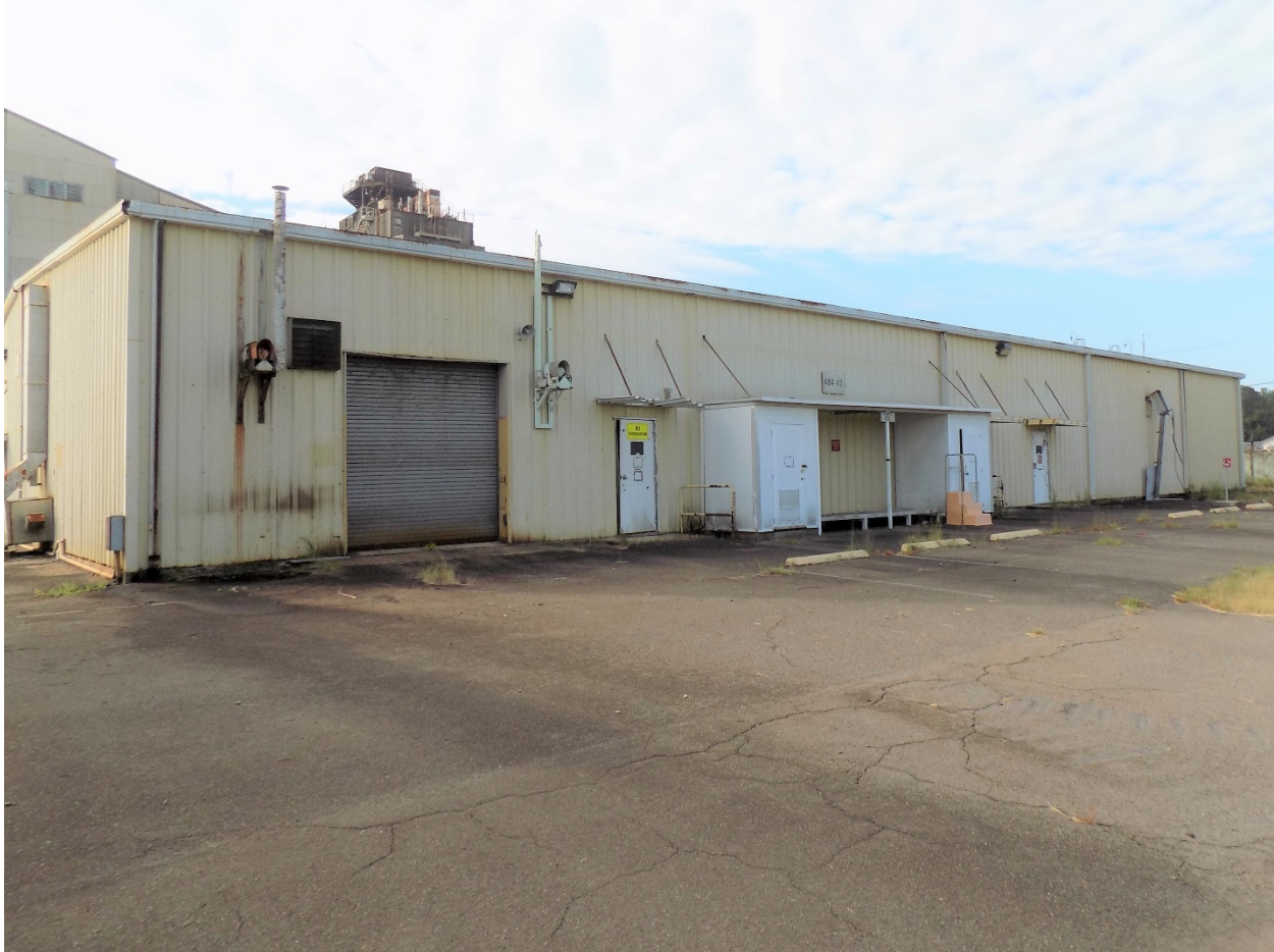
Figure 1: Building 484-4D Before
