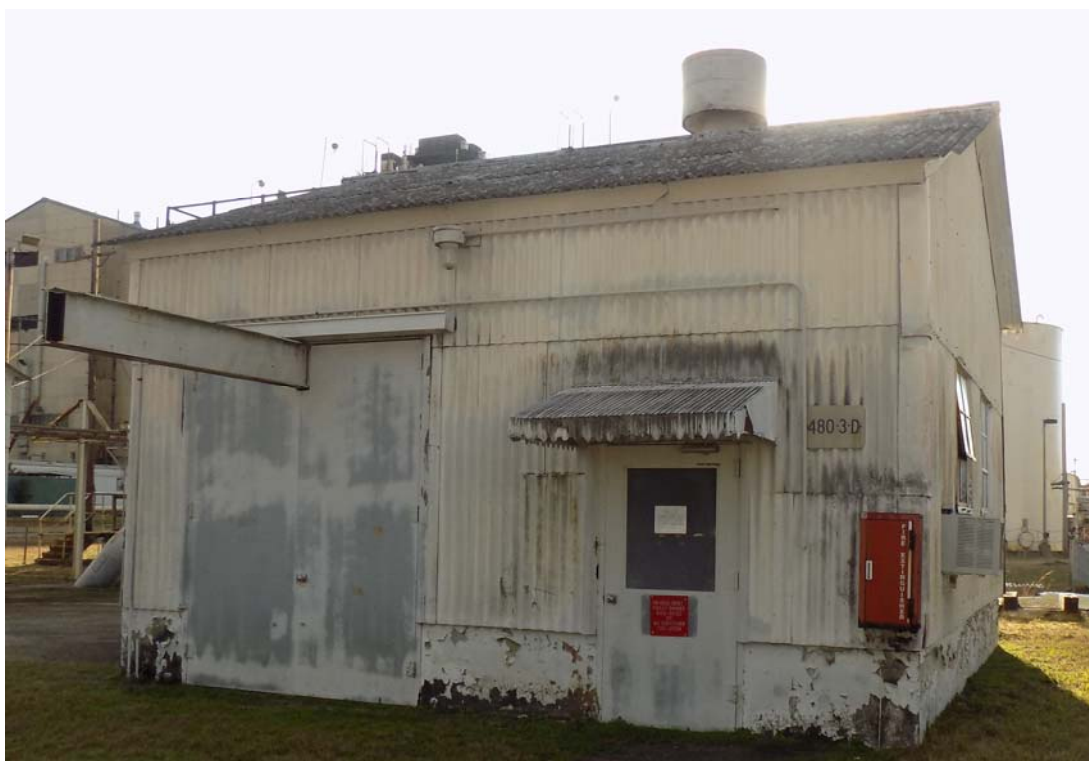
Figure 1. Photograph of Building 480-3D
