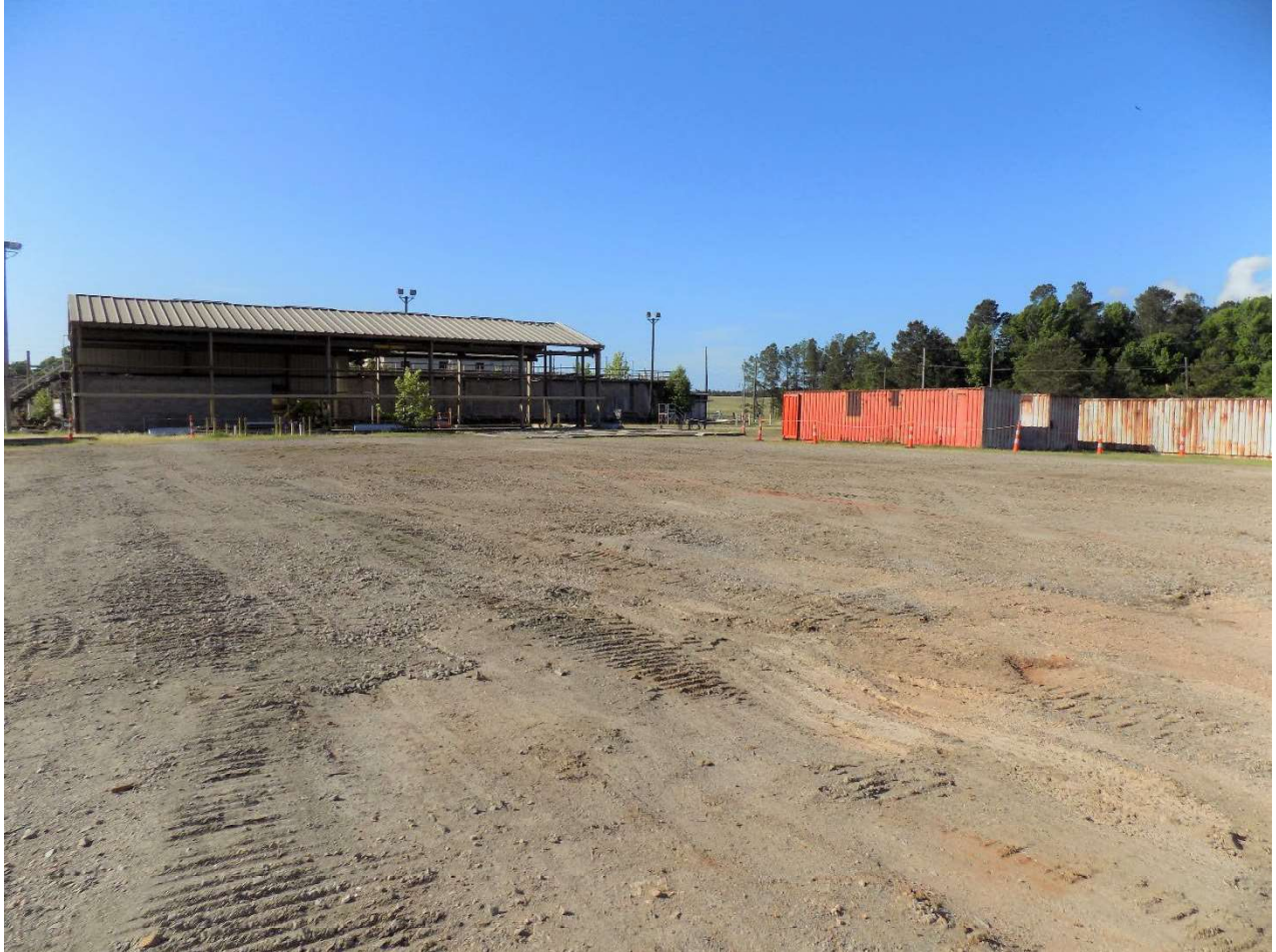
Figure 2. Building 704-7D (Looking Southwest) After Decommissioning
