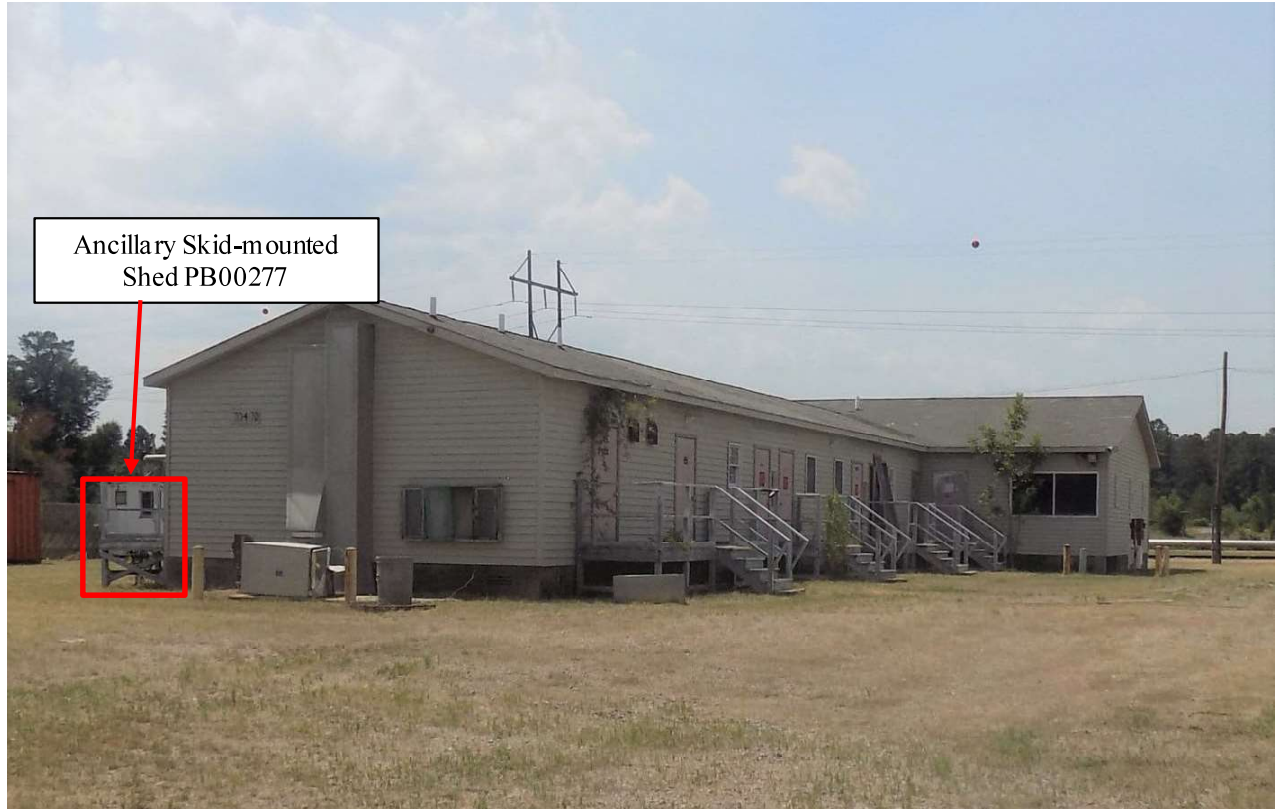
Figure 1. Building 704-7D (Looking Northwest) Before Decommissioning
