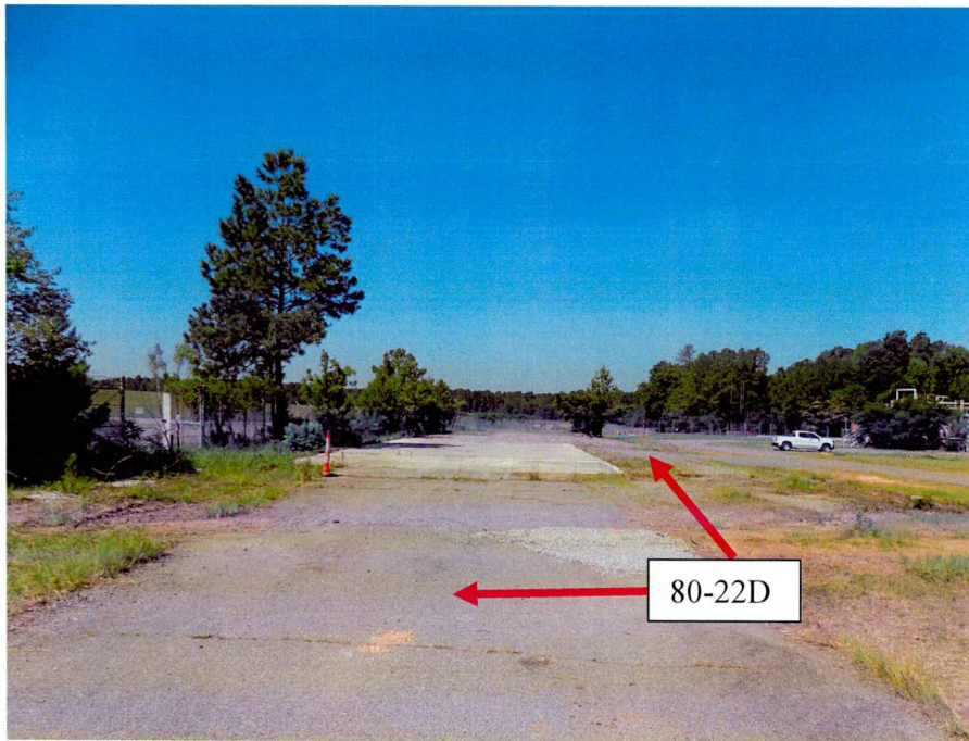
Figure A-2. 484-13D and 80-22D, (Looking Southwest) After Decommissioning
