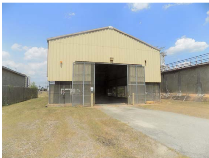
Figure 1. Building 683-D, Chlorine Unloading and Storage
