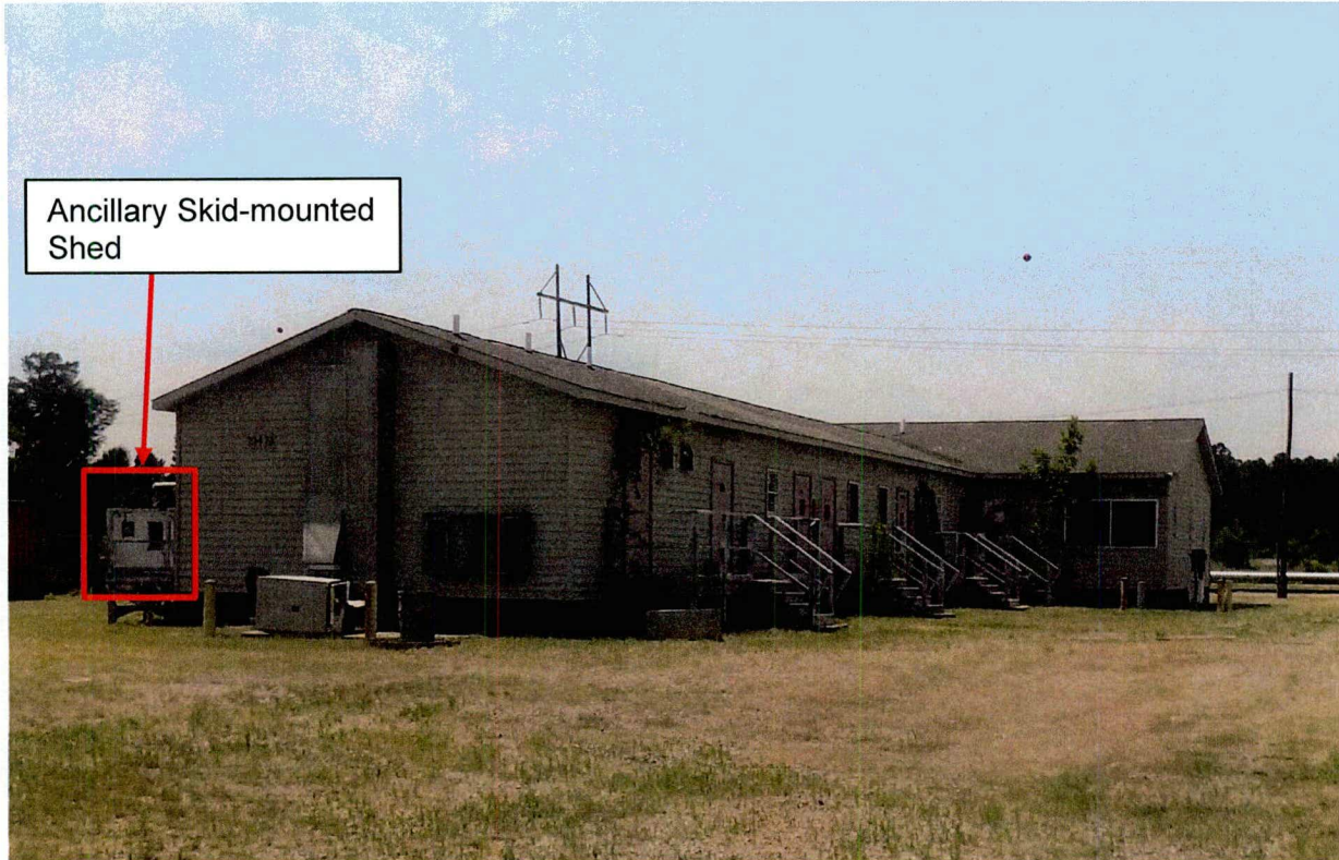
Figure 6. Building 704-7D, D-Area Maintenance Building
