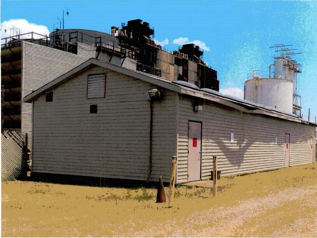
Figure 17. Building 717-3D, D-Area Welding Shop
