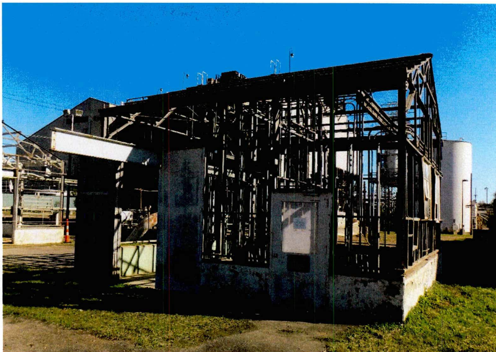
Figure 2. Building 480-3D, Maintenance Field Office and Shop
