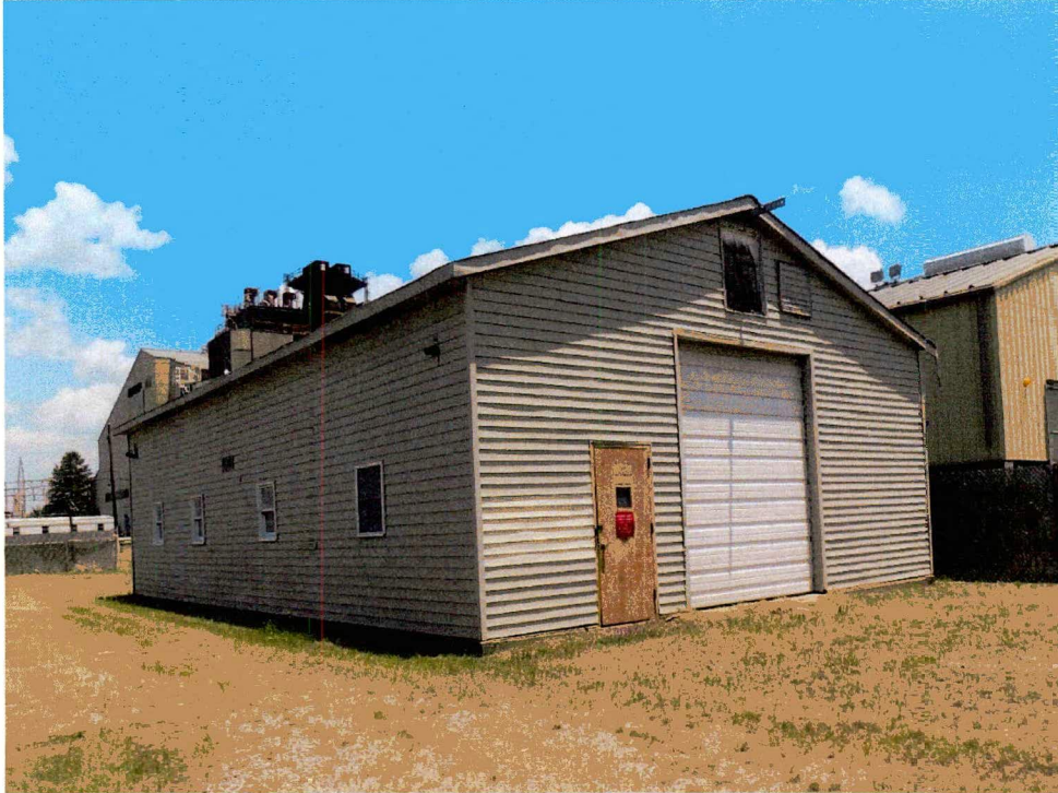
Figure 14. Building 710-16D, Storage Building
