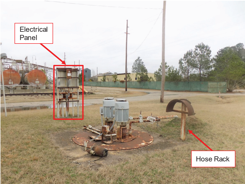
Figure 11. Sanitary Sewage Lift Station 607-12D (currently abandoned)
