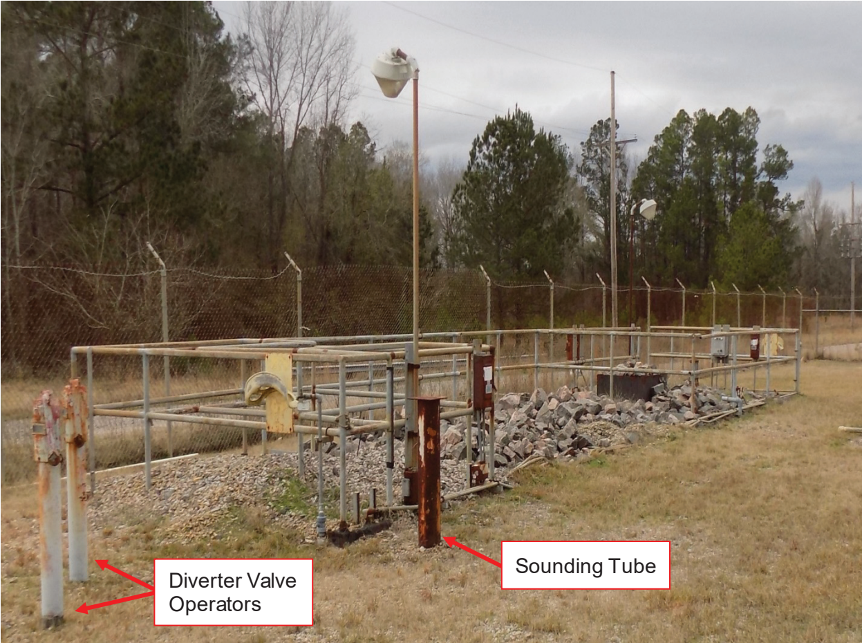
Figure 7. Building 607-15D, Sanitary Waste Treatment Plant
