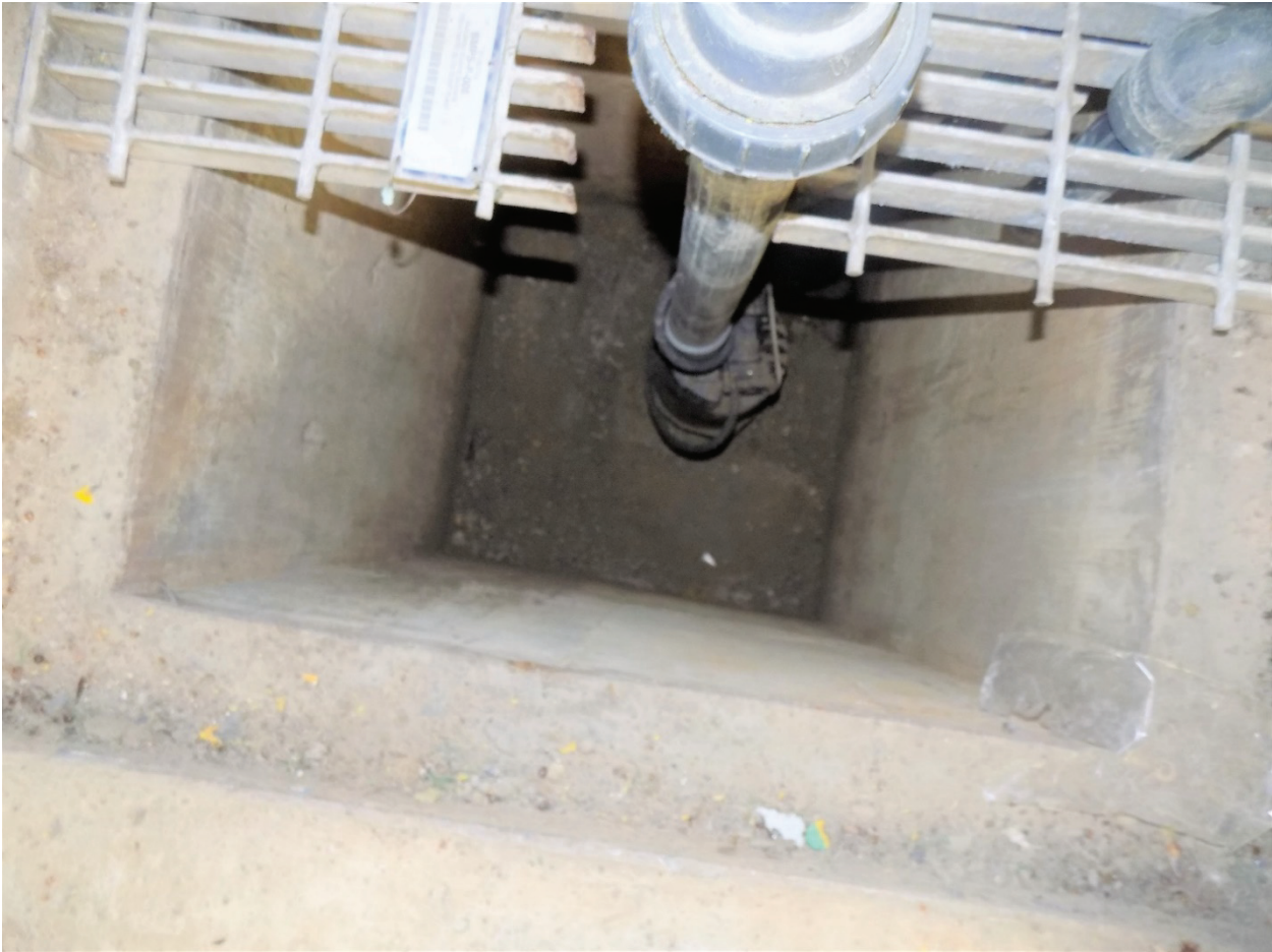
Figure 6. Building 607-14D Collection Sump
