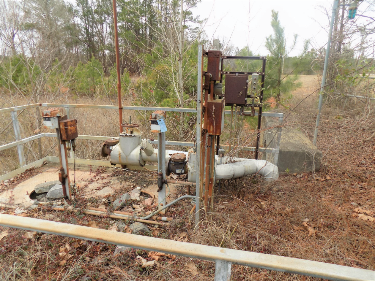
Figure 13. 483-6D Surge Basin Remnants
