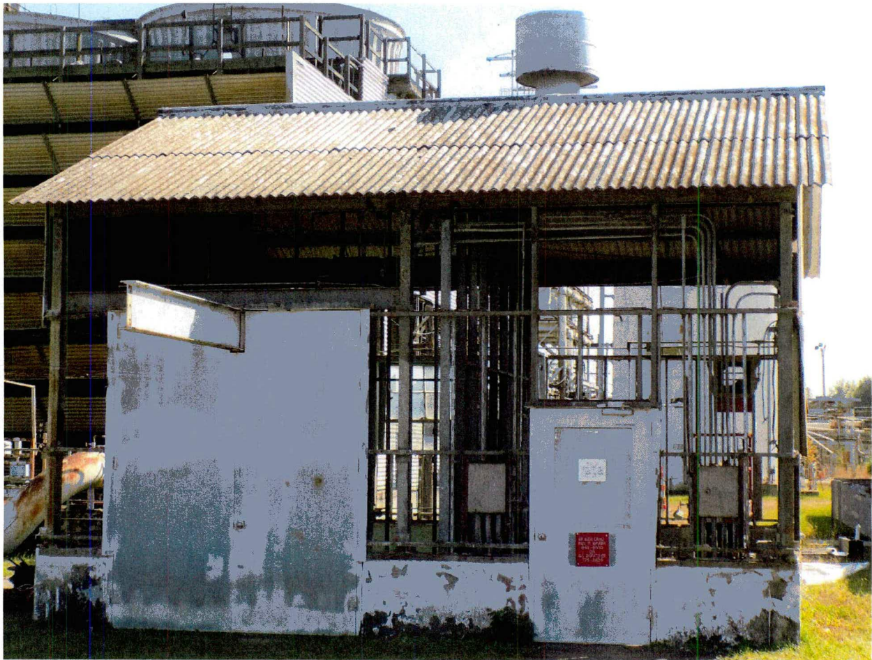
Figure 3: Photo Building 480-3D Looking South (North Side of Building)
