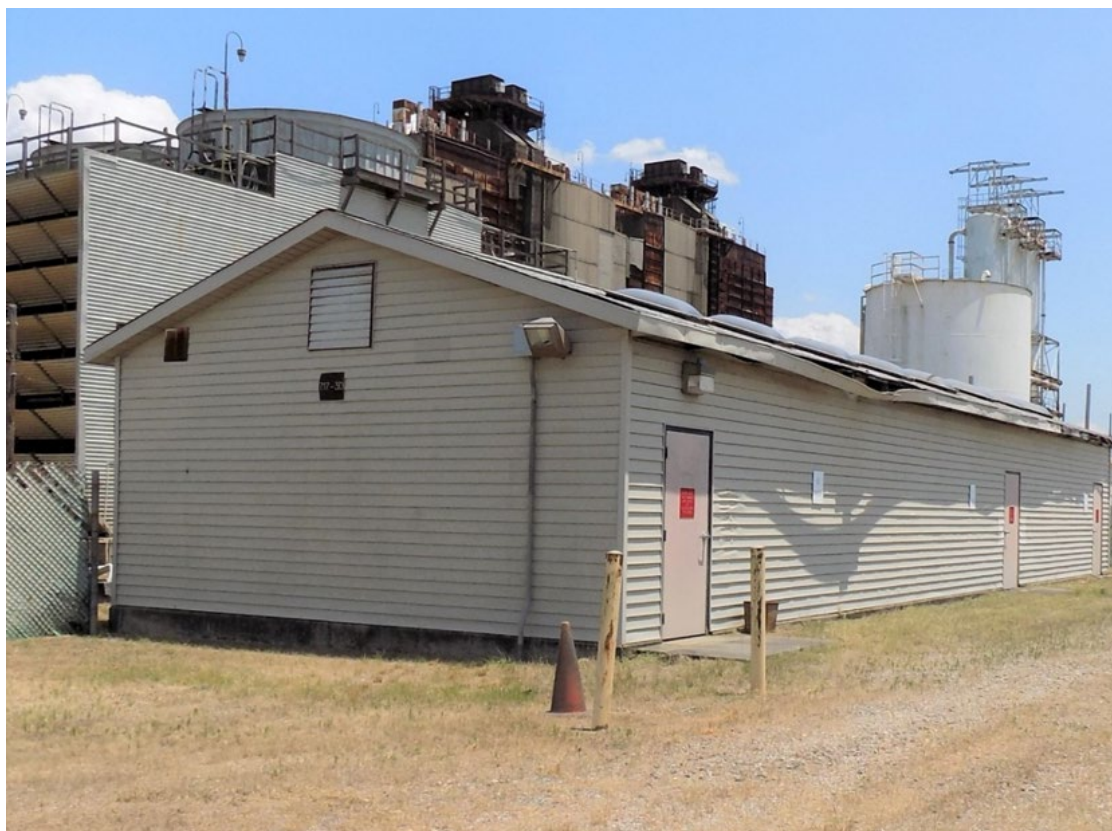
Figure A-1. Building 717-3D (Looking Southeast) Before Decommissioning
