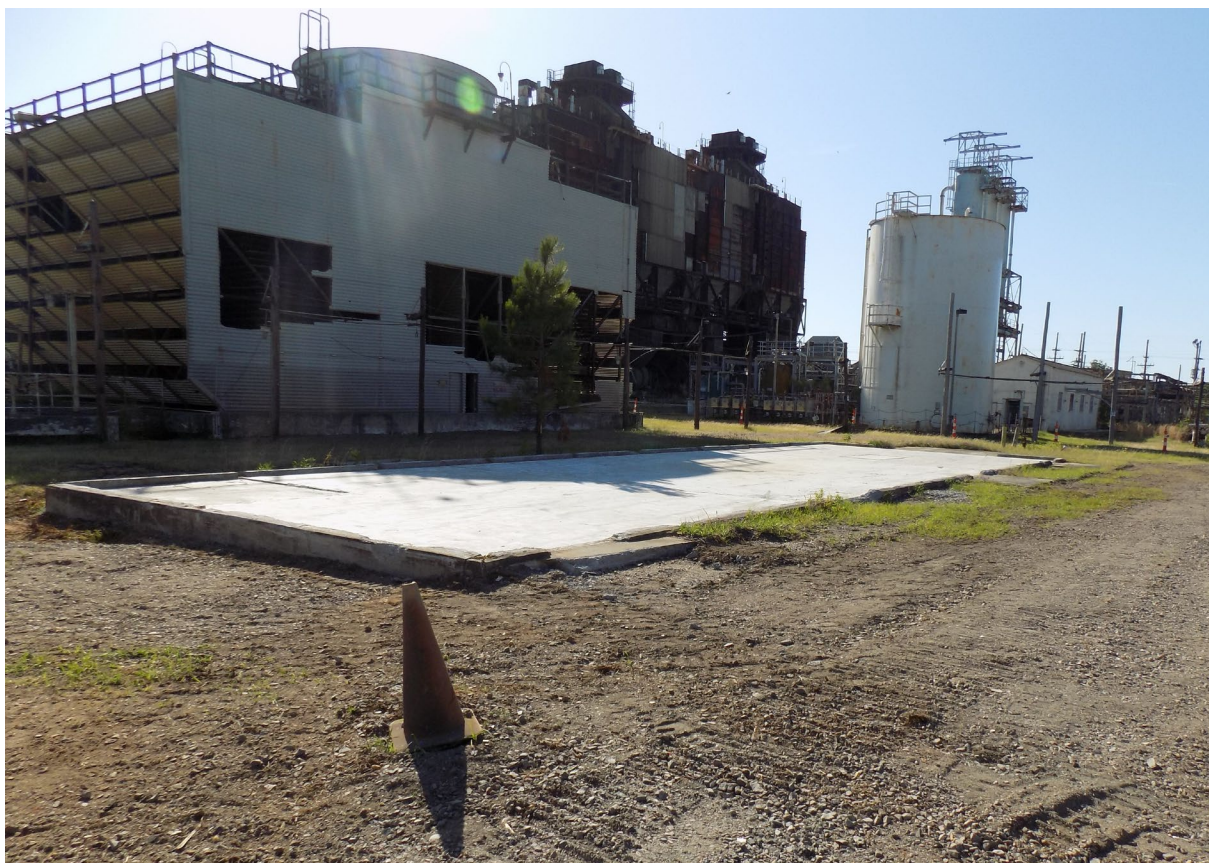
Figure A-2. Building 717-3D (Looking Southeast) After Decommissioning
