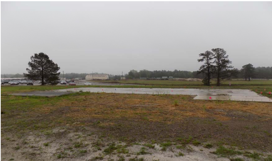
Photo 2 – Building 728-N, Shipping Cask and Railroad Car Repair Facility - After (Looking Southwest)
