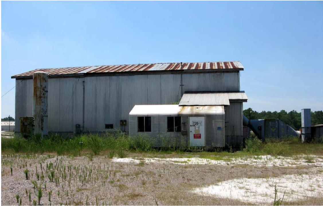
Photo 1 – Building 728-N, Shipping Cask and Railroad Car Repair Facility - Before (Looking Southwest)
