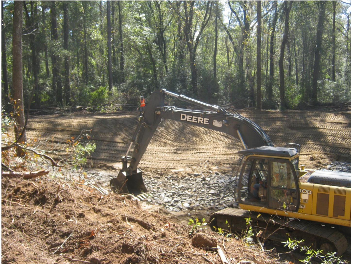
Figure 9. Structural Stone Prior to Common Fill
