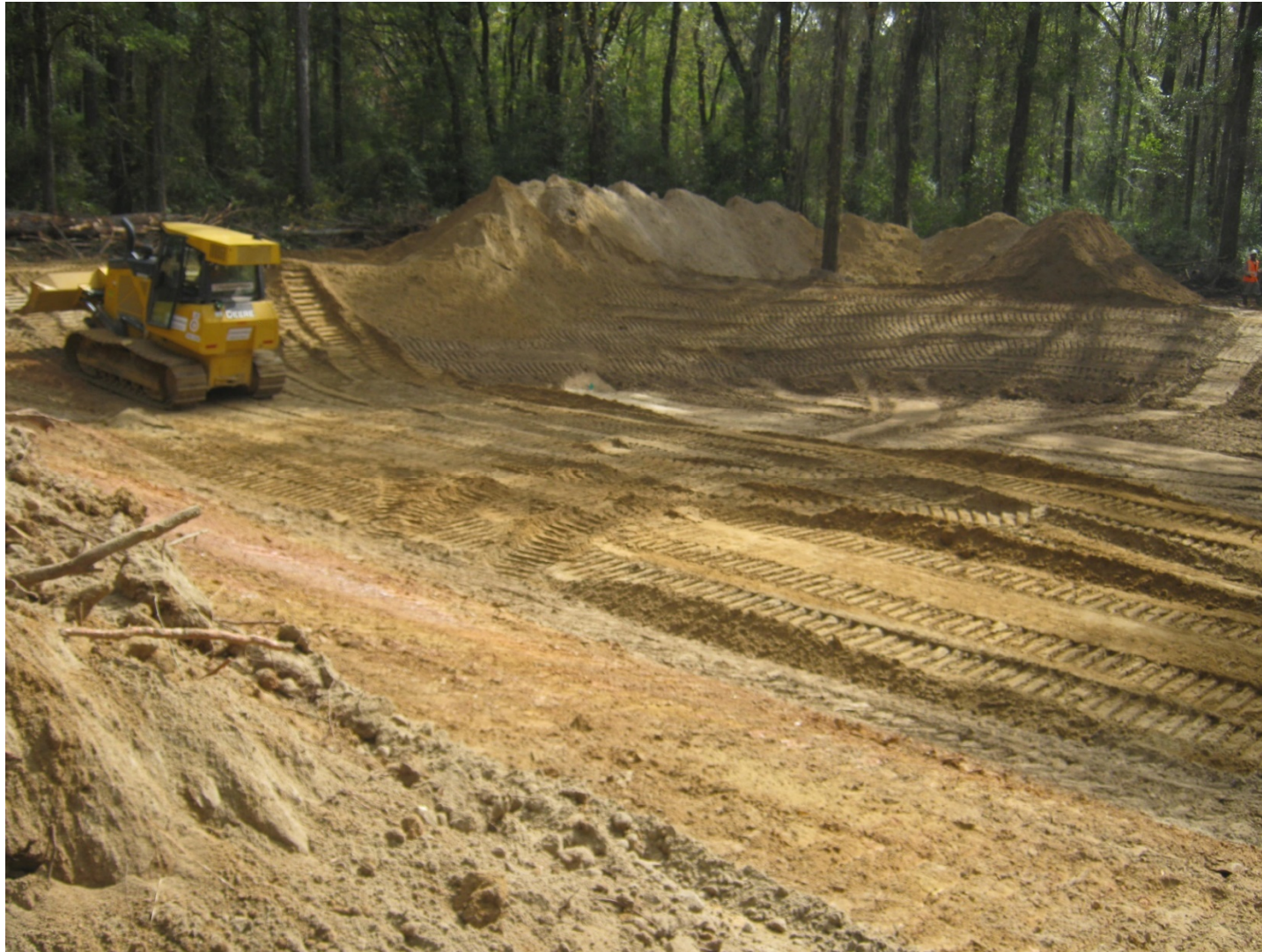
Figure 10. Placement of Common Fill in Support of GOSB OU Closure
