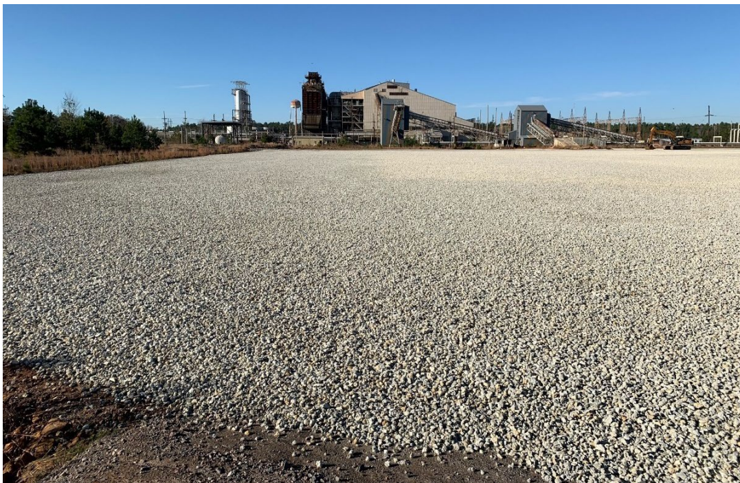
Photo 7. Finished Limestone Gravel Cover
