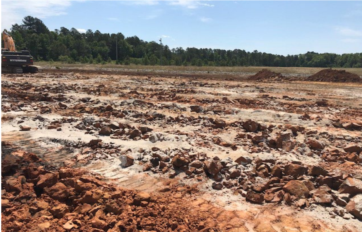
Photo 3. Amendment Spread over Decompacted Soils
