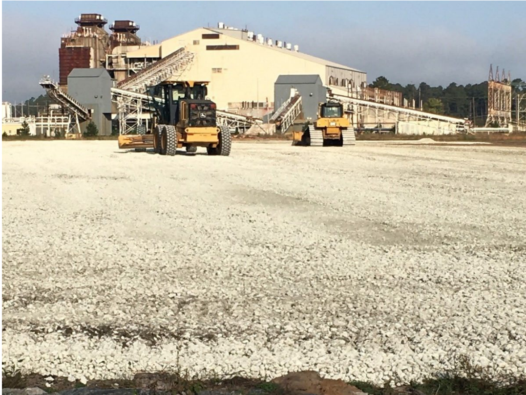
Photo 6. Placement of Limestone Gravel Stabilization
