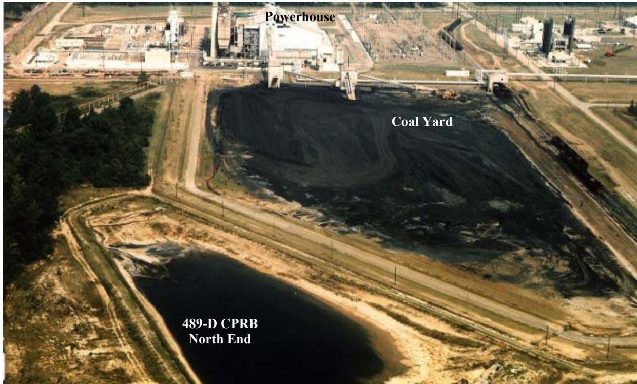
Photo 1. Historical Photo of D Area (1982)
