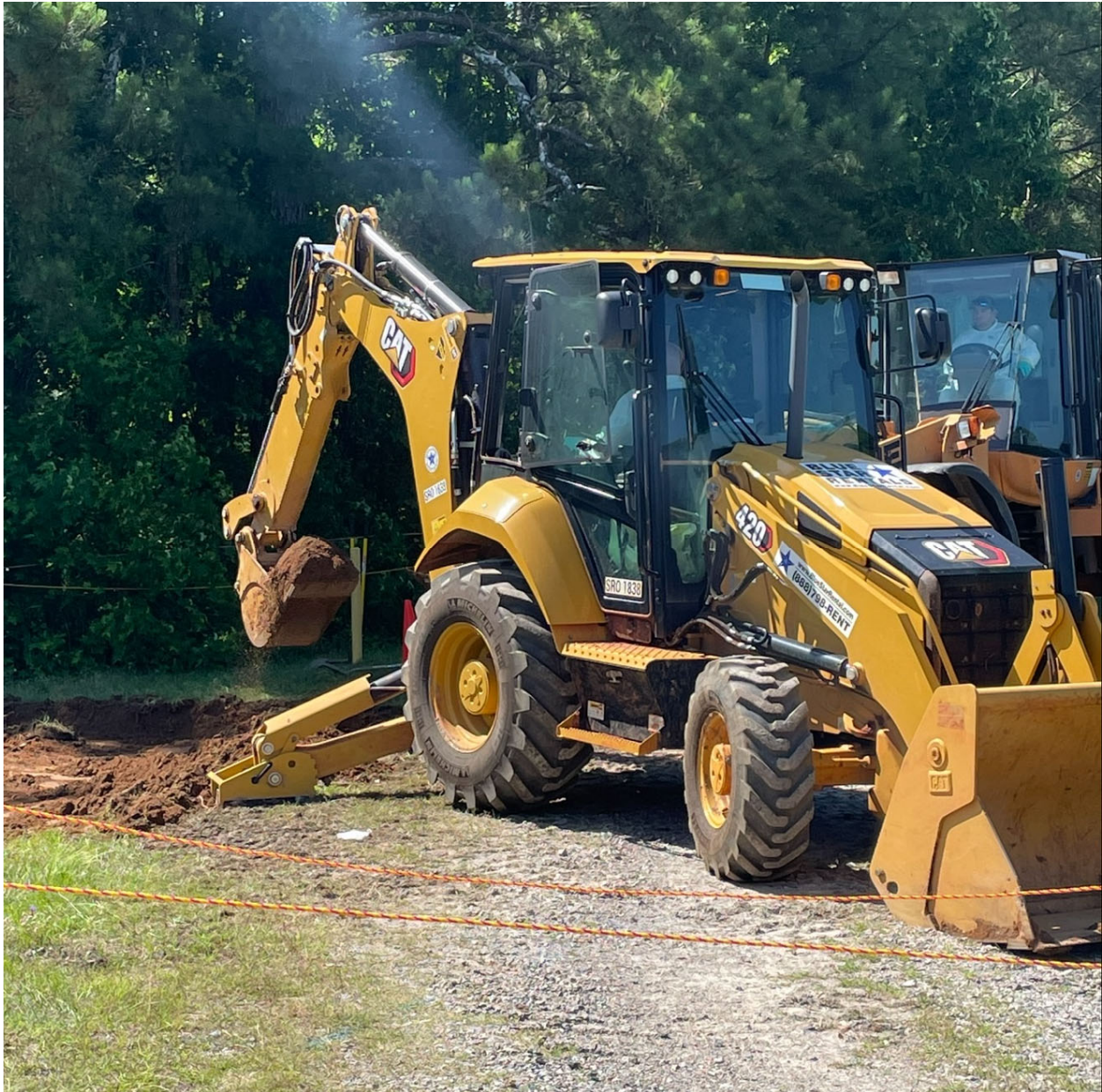
Figure 6. Equipment Used for the 904-44G Spill Release Area Soil Excavation (2024)
