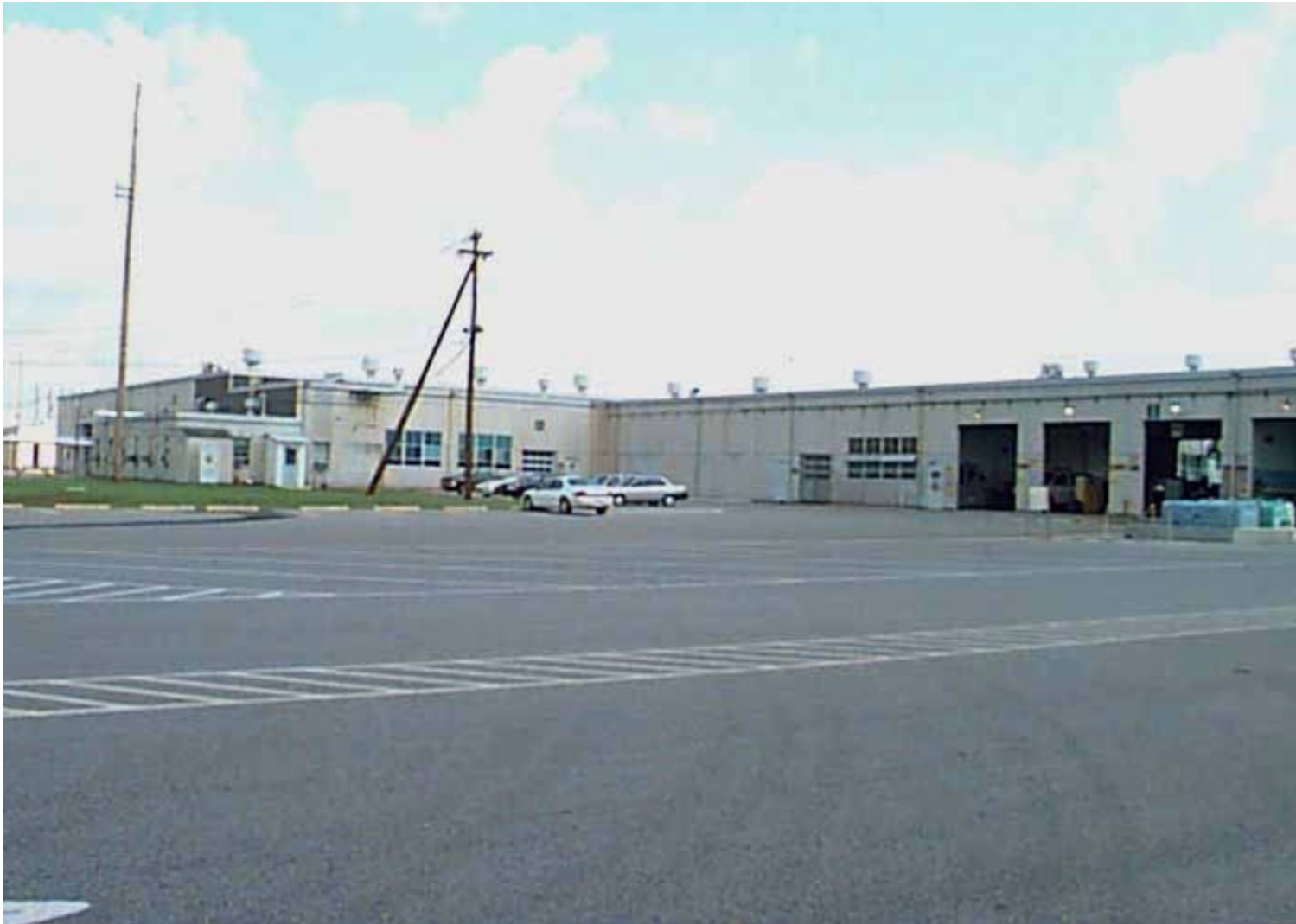
Figure 4. Automotive Repair Shop (716-A) OU Before Decommissioning
