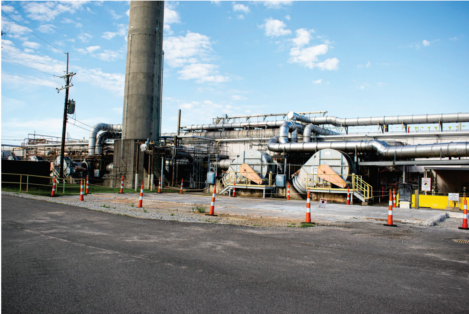
Figure 4: 236-H Looking Southwest (After)
