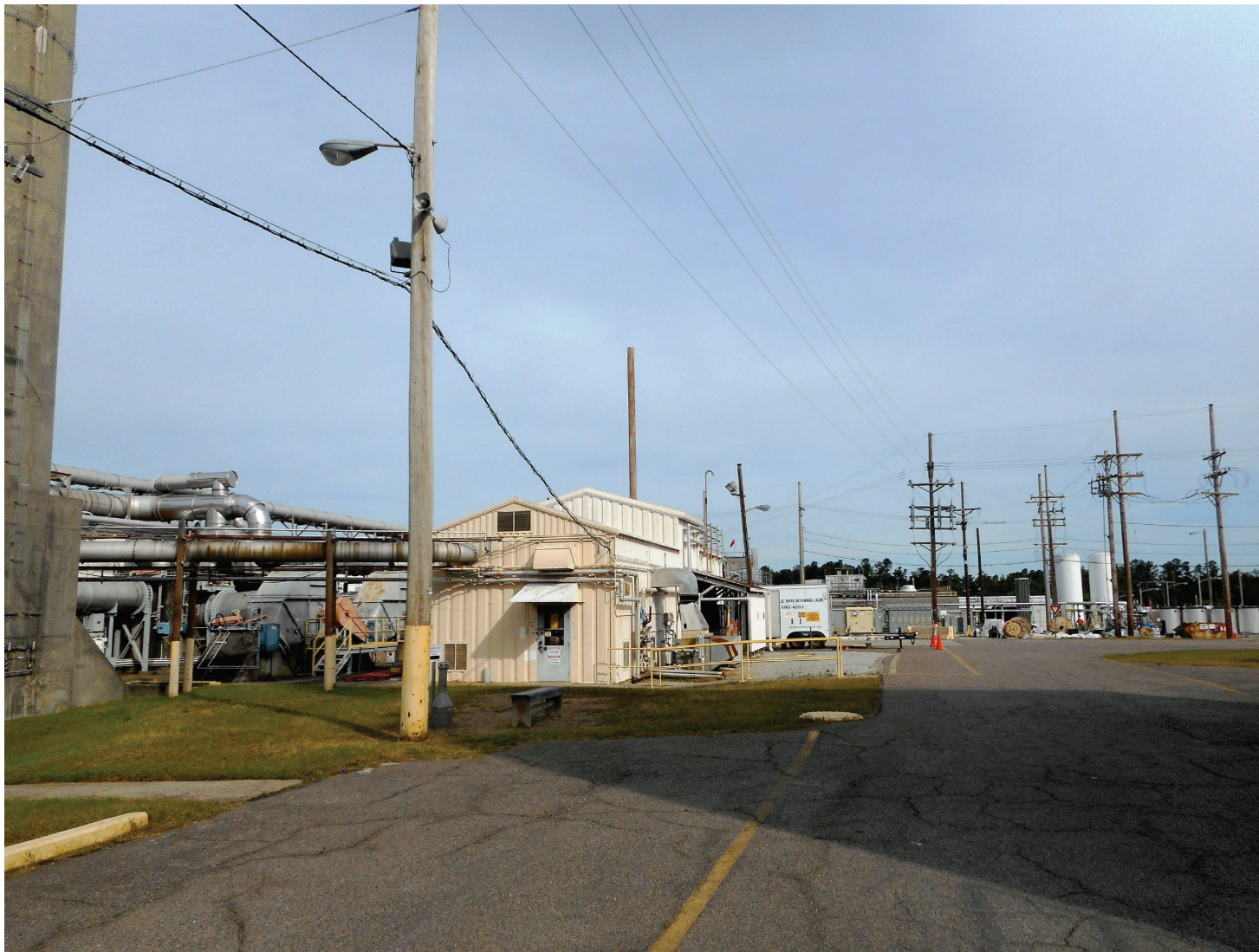
Figure 2: 236-H Looking Northwest (Before)
