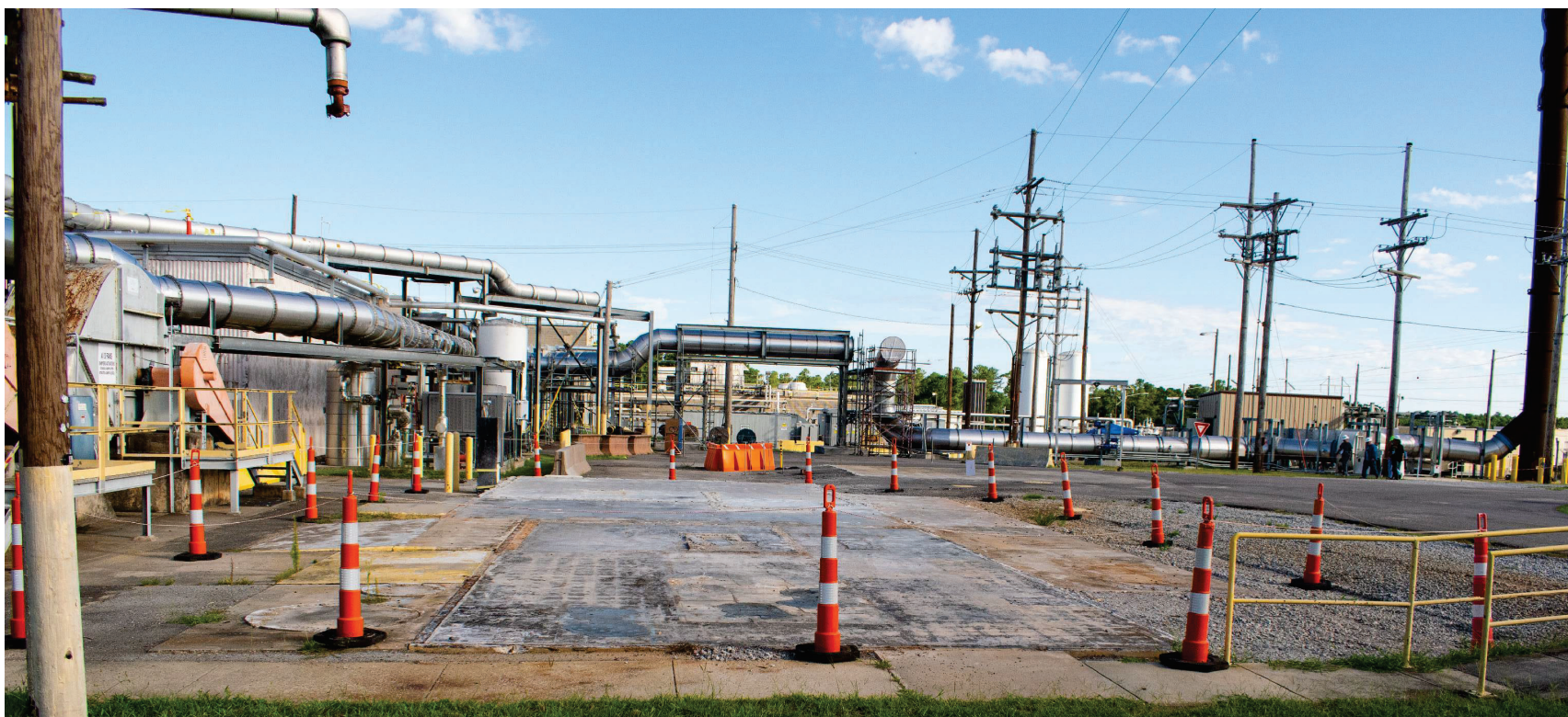
Figure 5: 236-H Looking Northwest (After)
