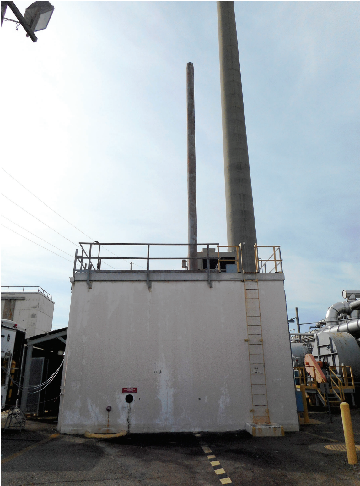
Figure 3: 236-H Looking Southeast (Before)
