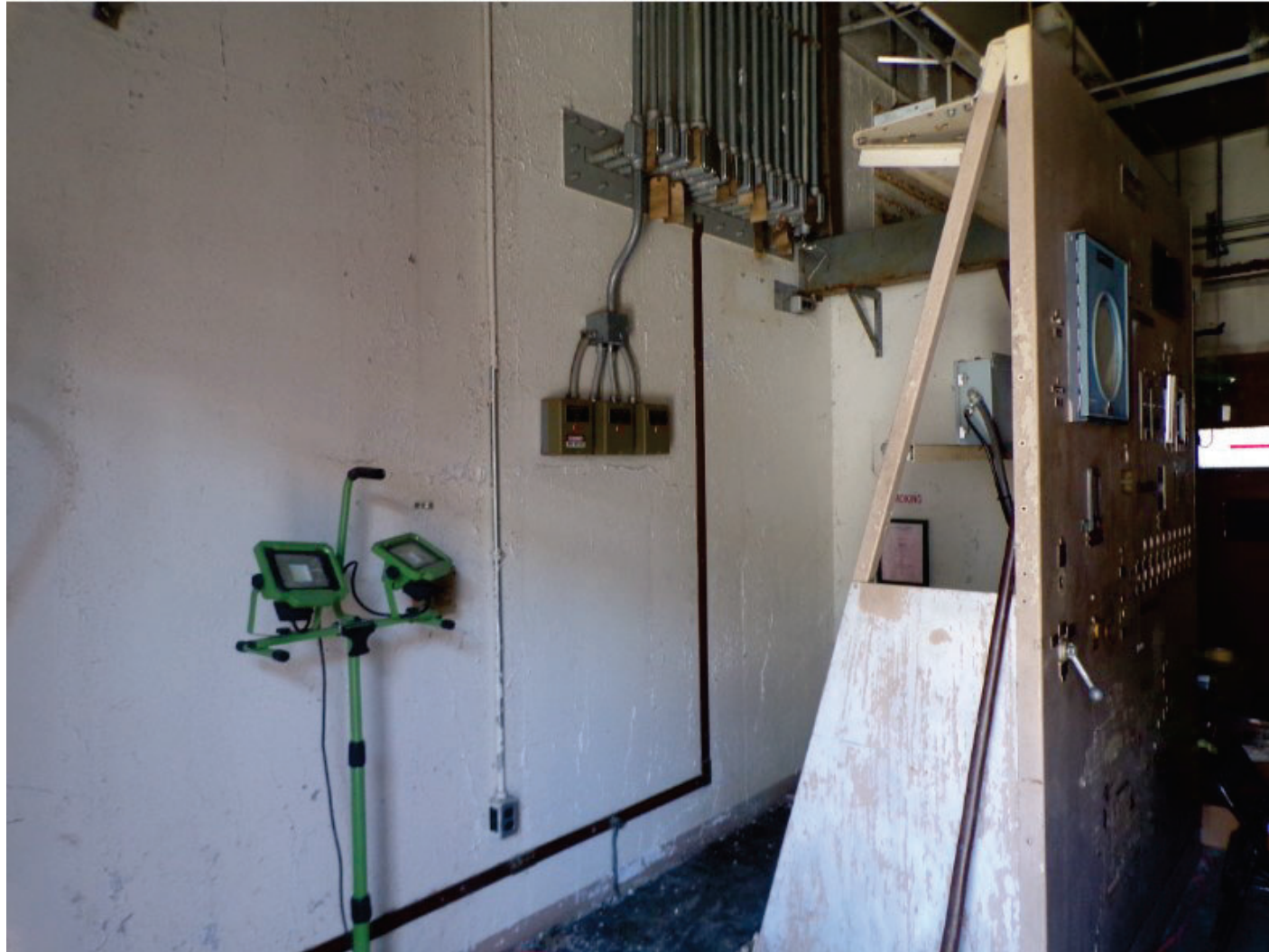
Figure 6. Back of Control Room Post Deactivation
