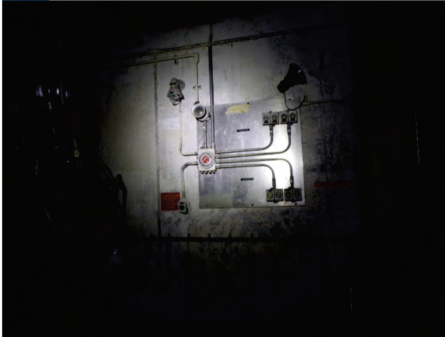
Figure 7. Alarm Panel Post Deactivation
