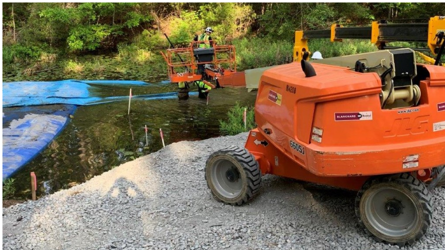
Figure 10. Photos of Equipment - Telehandler
