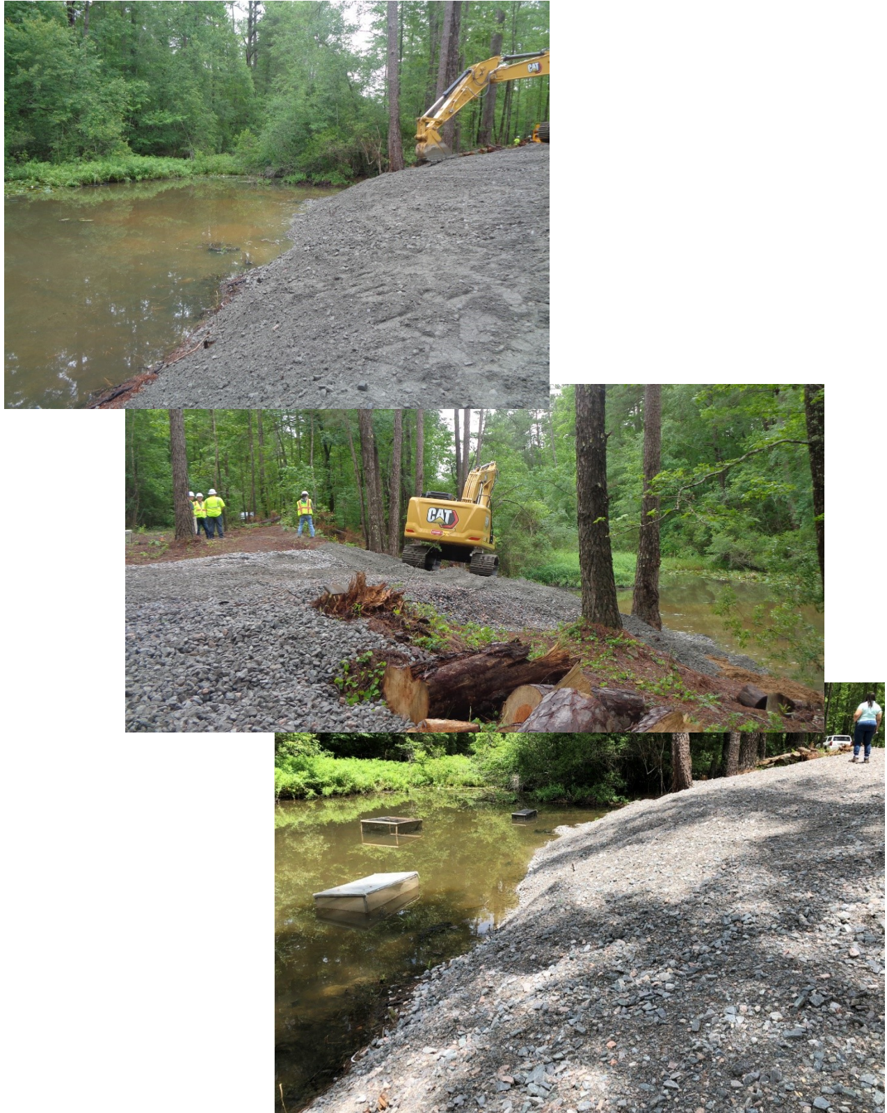
Figure 18. Final Grading and Final Acceptance Inspection
