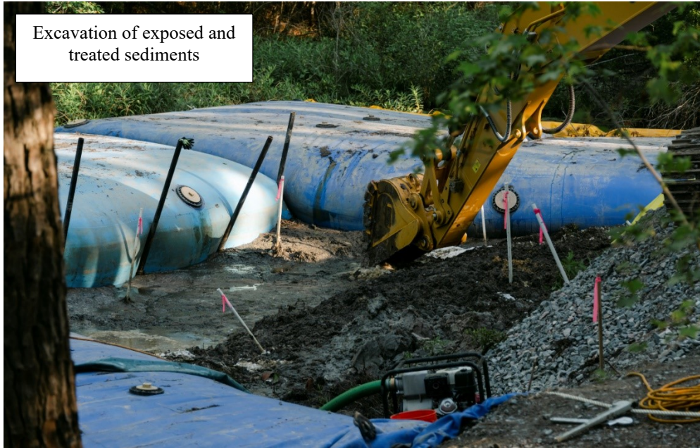
Placement of sediments in 1 cy double line sacks
