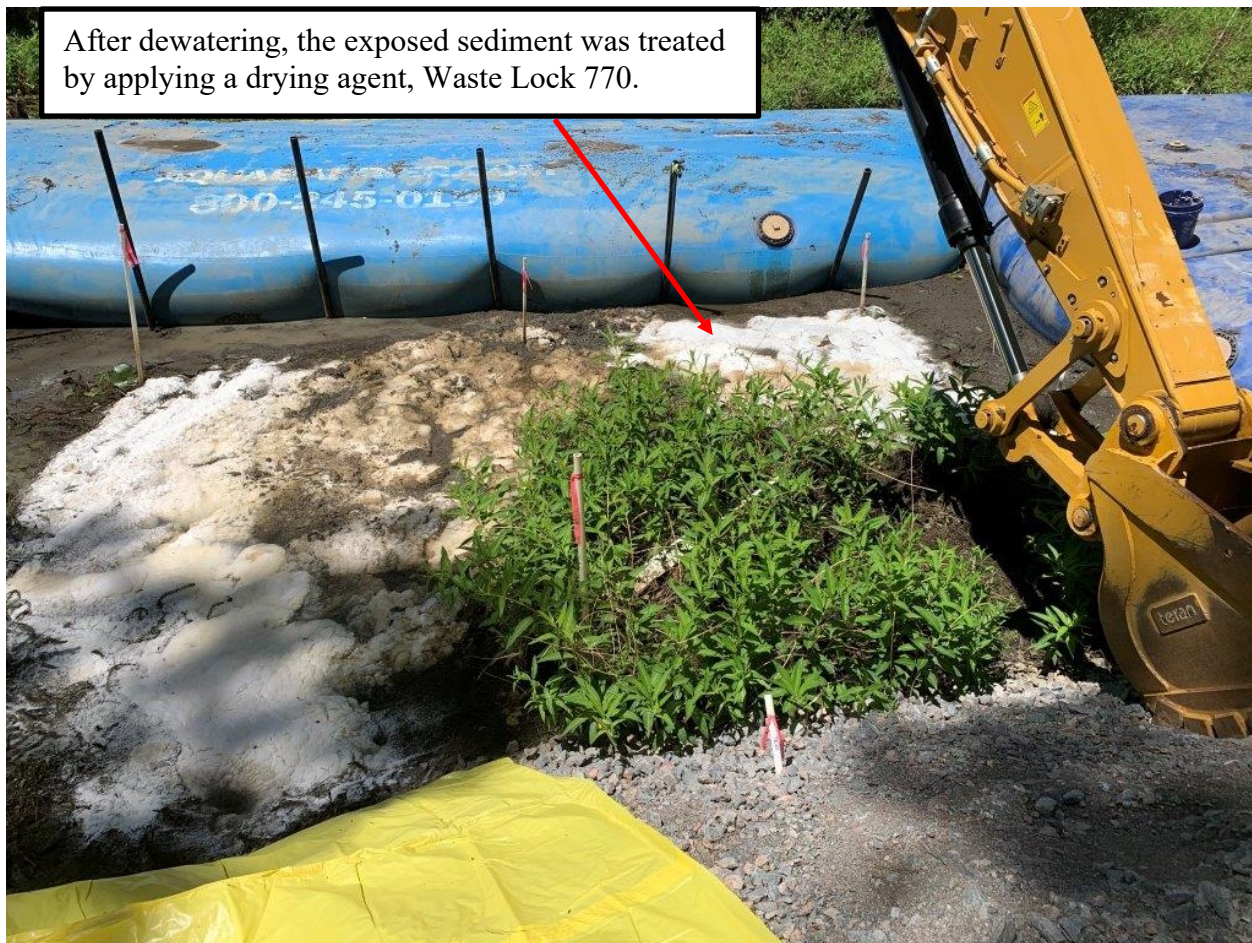
Figure 14. Dewatering of Excavation Area and Treatment of Sediments
