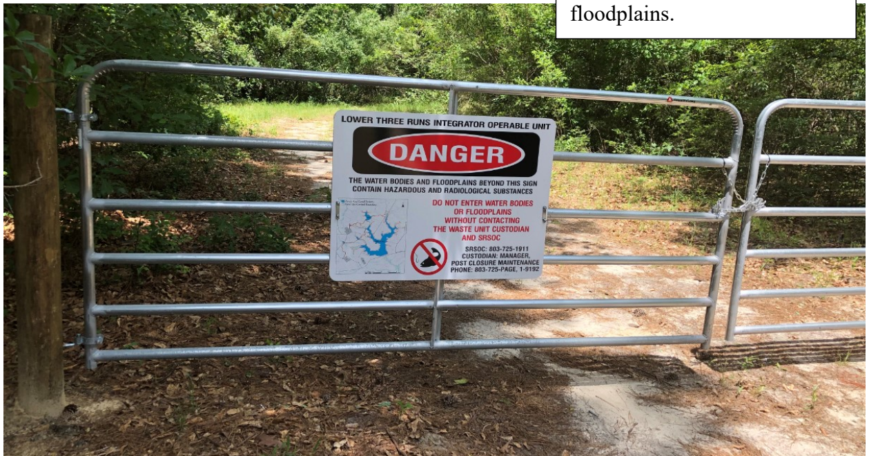
Figure 20. Access Control Warning Signs (typical)
