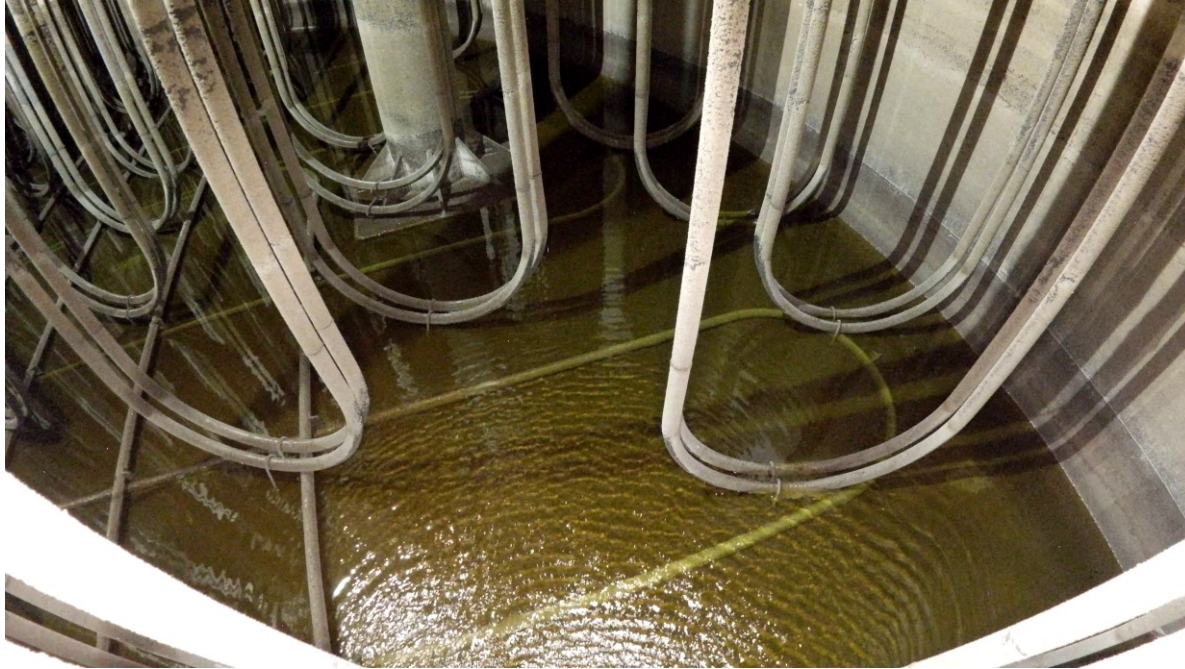
South Tank Wall
