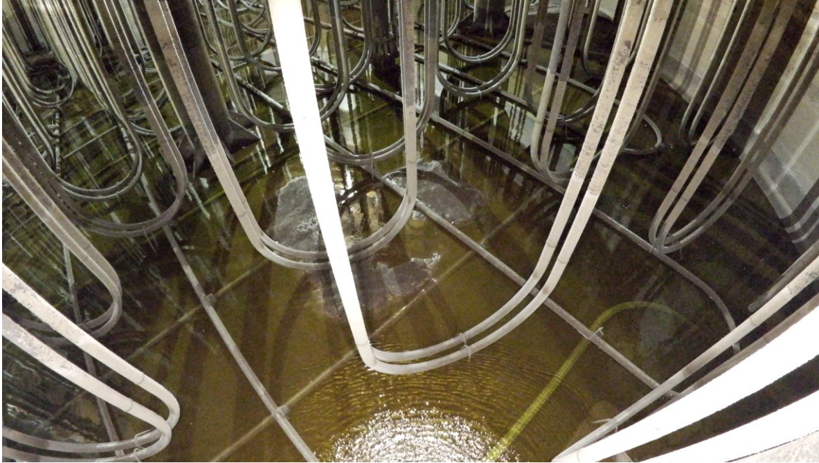
Accumulation Below Riser 5
