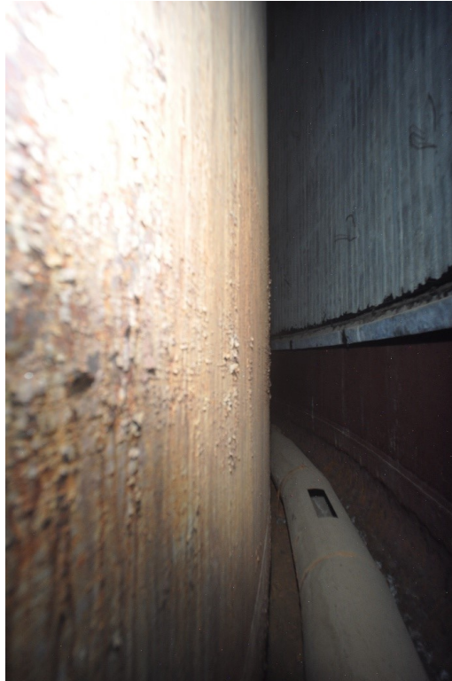
North Riser Facing West
