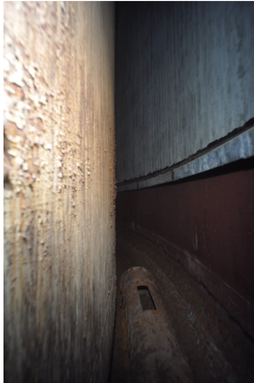
East Riser Facing North
