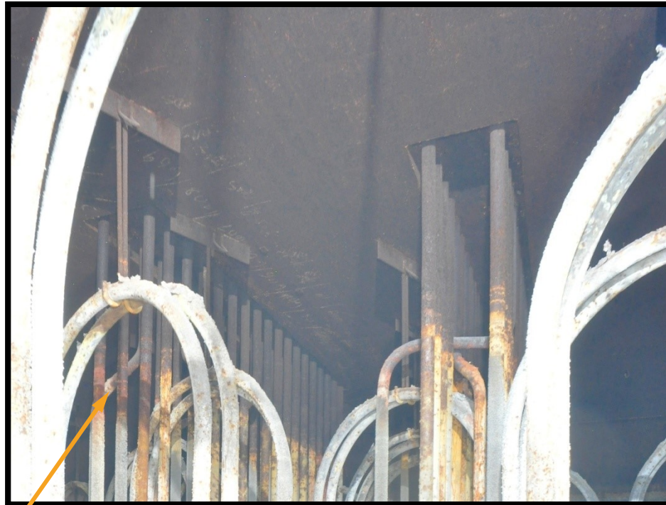
Cooling coil lines entering and exiting waste tank
