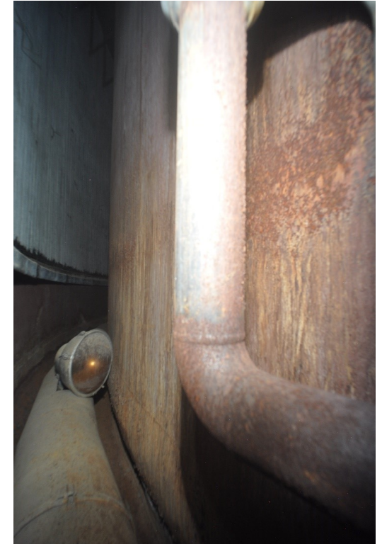
South Riser Facing West
