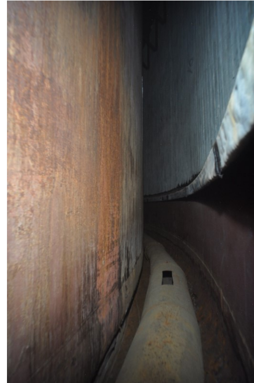
South Riser Facing East
