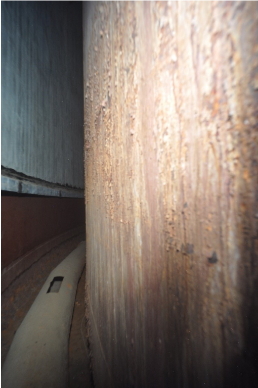
North Riser Facing East
