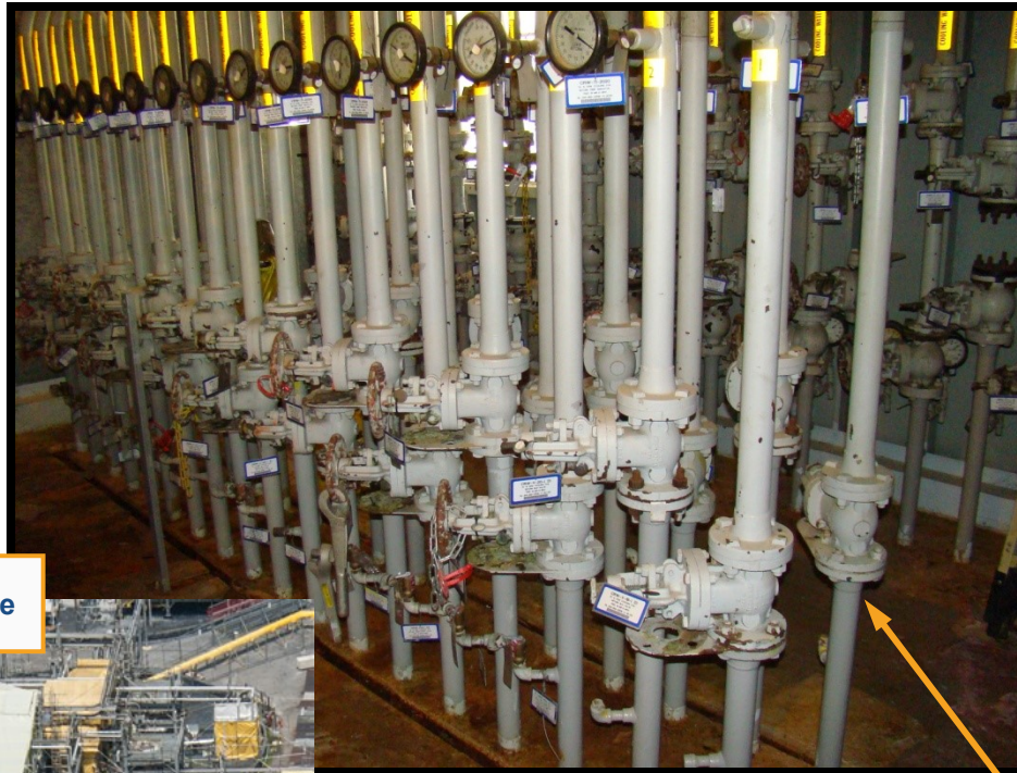
Cooling coil lines entering and exiting waste tank
