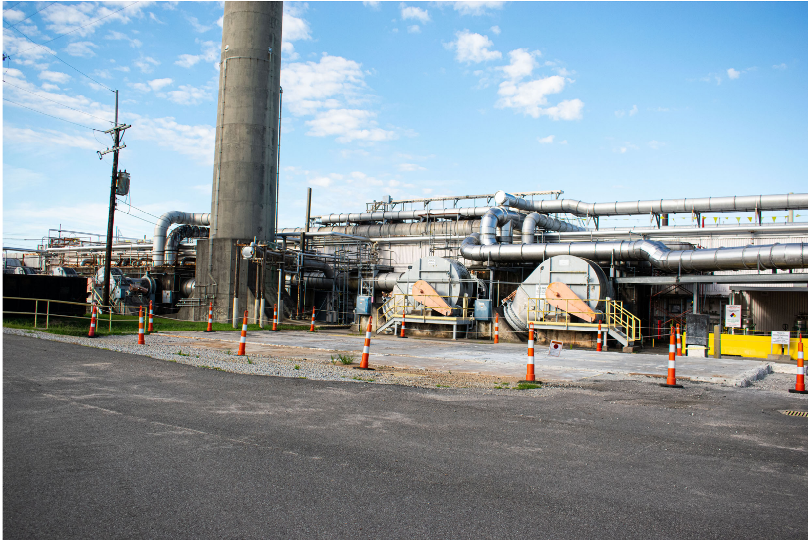
Figure 4. 236-H Looking Southwest (After)
