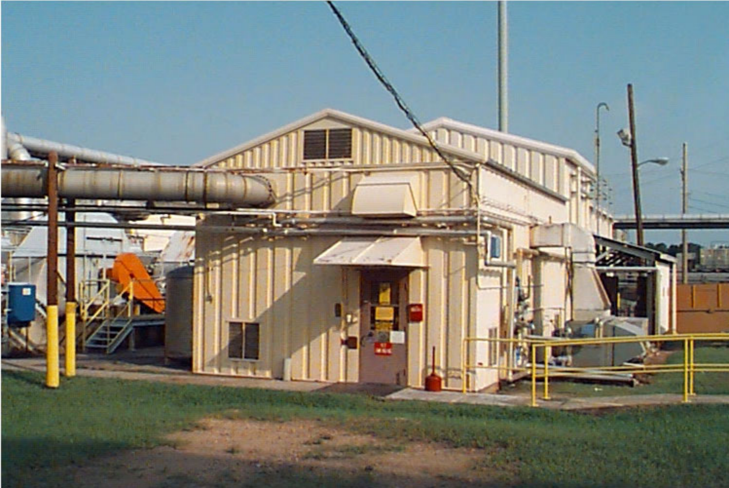
Figure 3. Ground View of South Section of the 236-H By-Product Purification Facility
