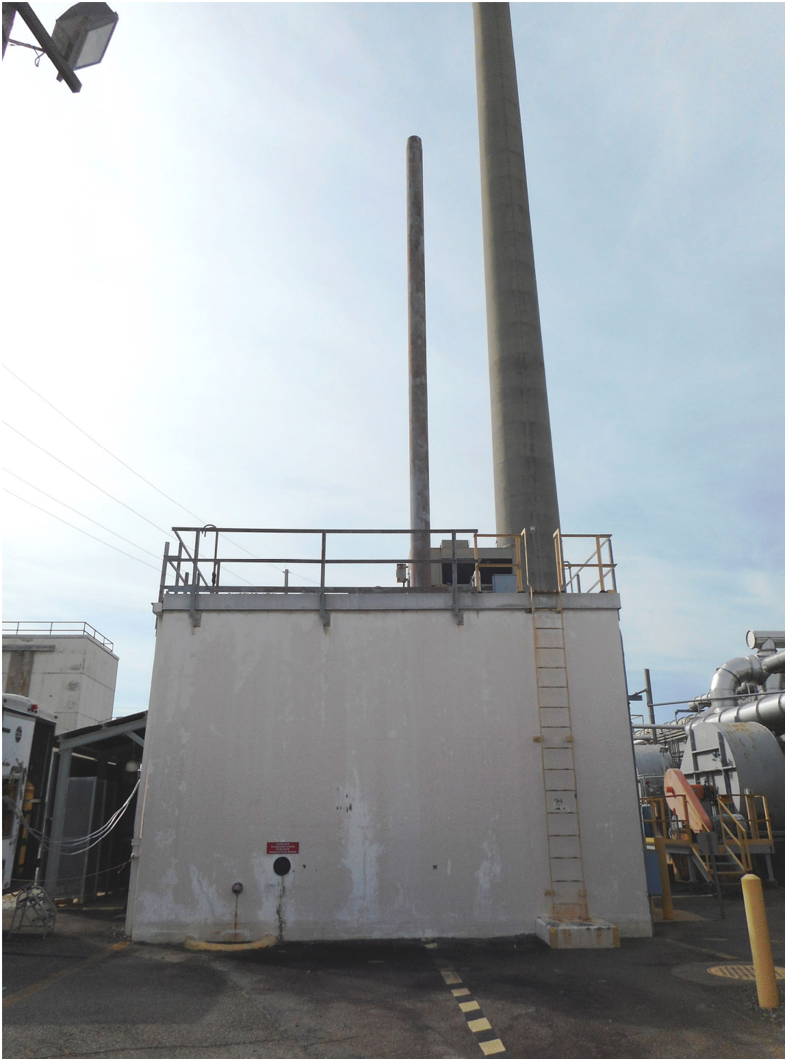
Figure 3. 236-H Looking Southeast (Before)
