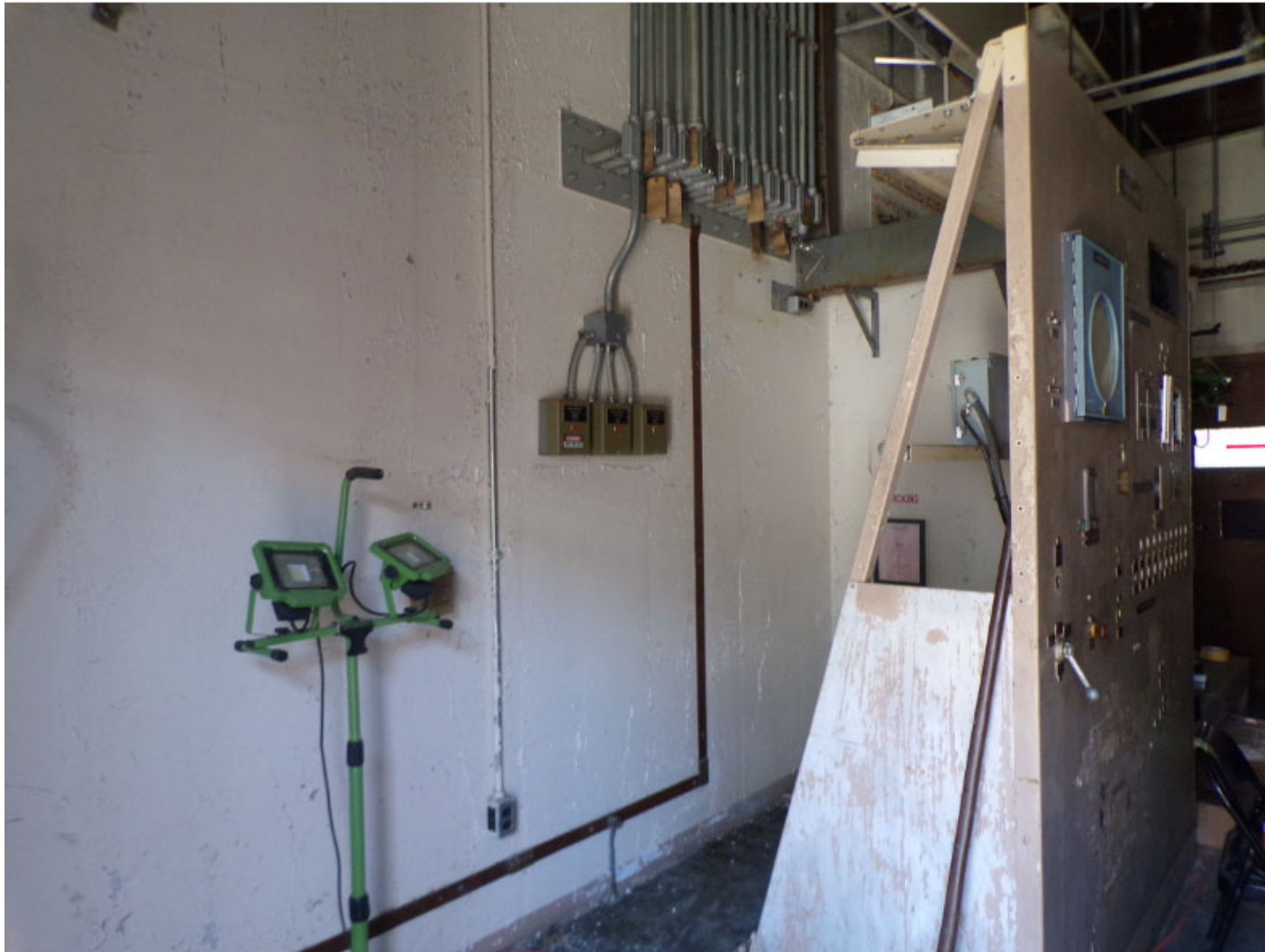
Figure 6. Back of Control Room Post Deactivation
