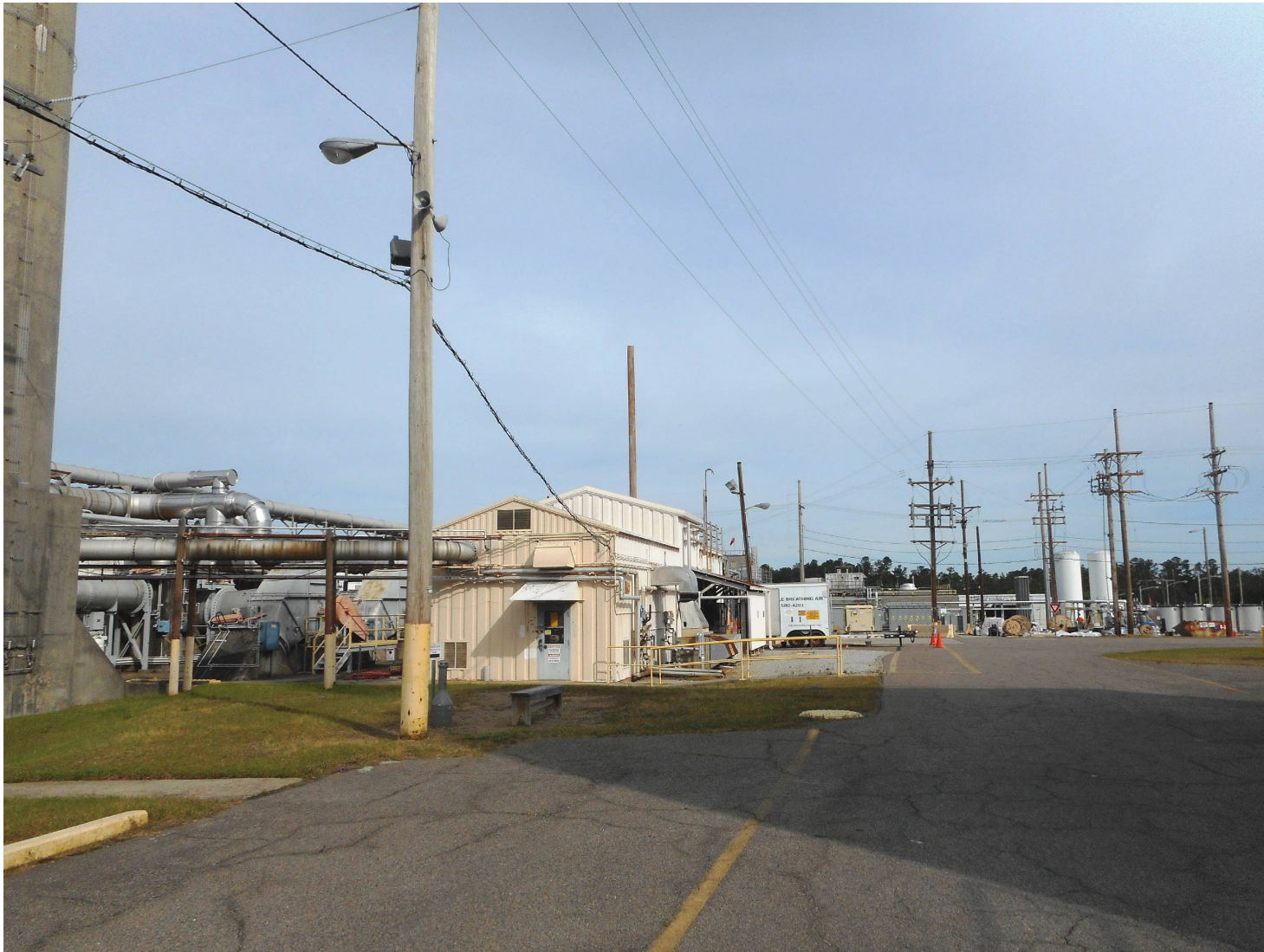
Figure 2. 236-H Looking Northwest (Before)
