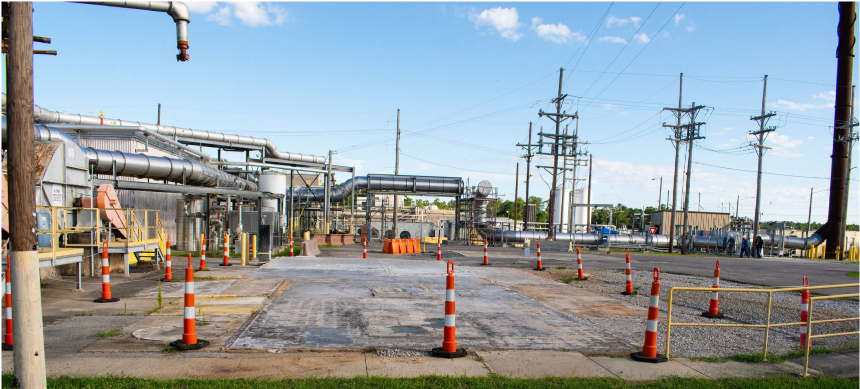
Figure 5. 236-H Looking Northwest (After)
