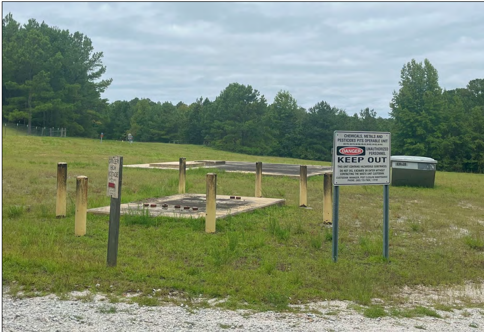
Figure D-5. Photo of CMP Pits (Current) (2024)
