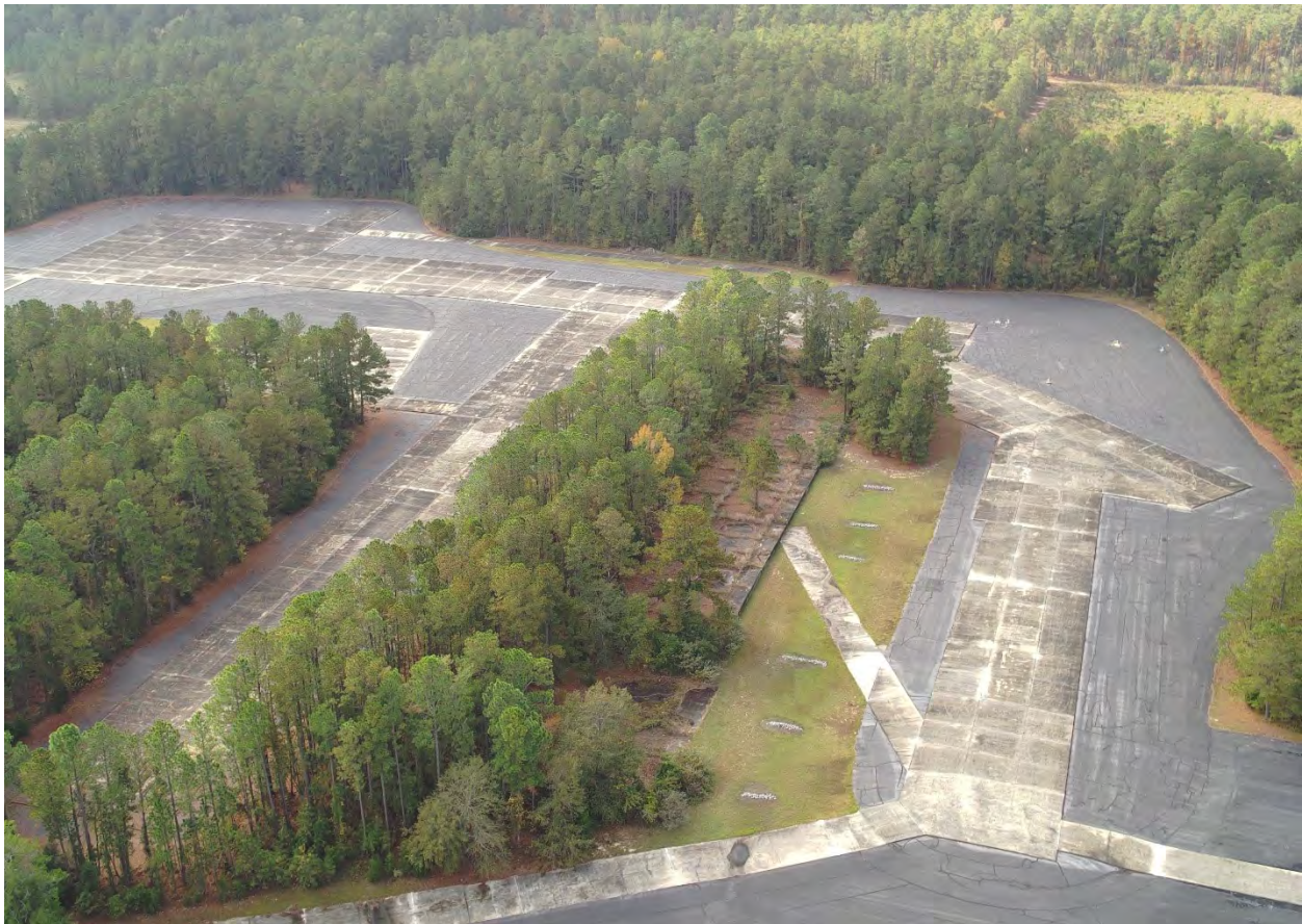
Figure H-5. Current Photos of the R-Reactor Seepage Basins OU (2024)
