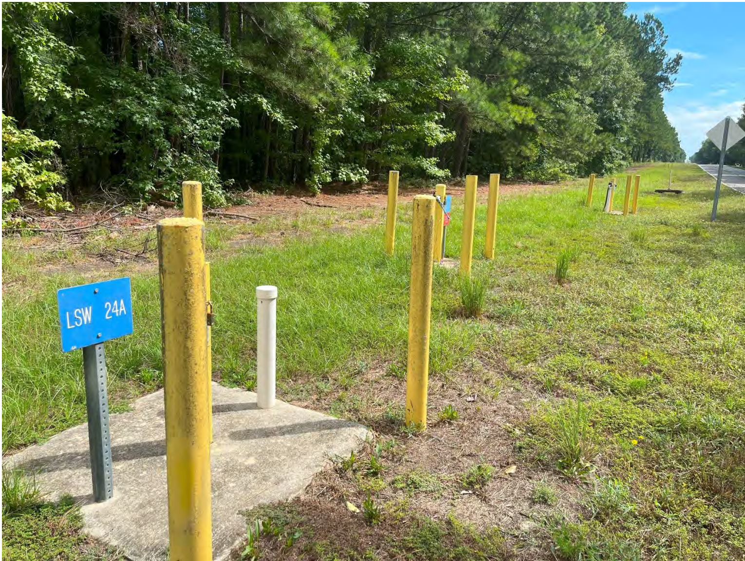
Figure F-5. Current (2024) Photo of LASG OU Monitoring Wells
